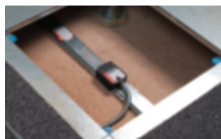
Electrak busbars
