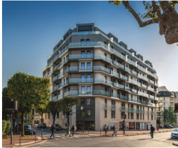
BNP Paribas Issy-Les-Moulineaux 60 connected apartments
